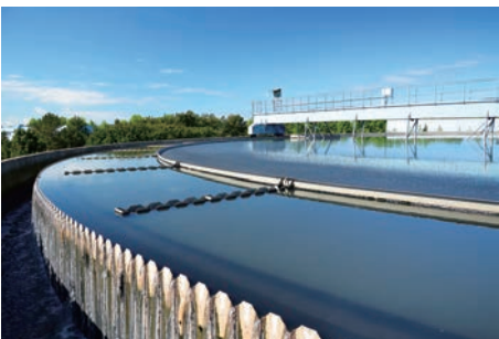
医药中间体及高盐化工废水处理行业 High salt chemical wastewater treatment
